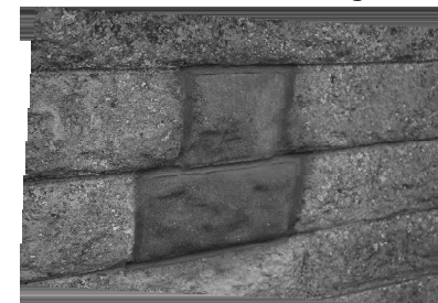
Making good the gas heater flue holes
